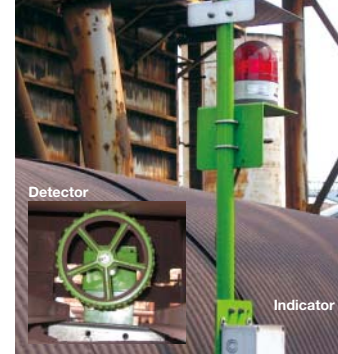
Conveyor Starting Indicator
