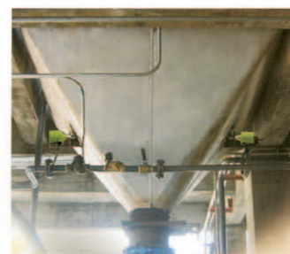
Microwave Barrier Switch for lower limit detection of Dust hopper
