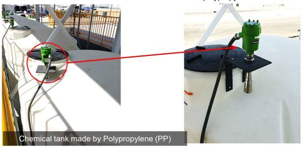
\*Picture: Radar transmitter installed at the outside of the polypropylene tank measures the chemical level.
